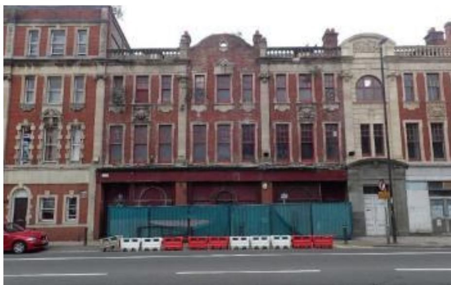
FIGURE 22: RESTORATION WORK TO GRADE II LISTED BUILDING
