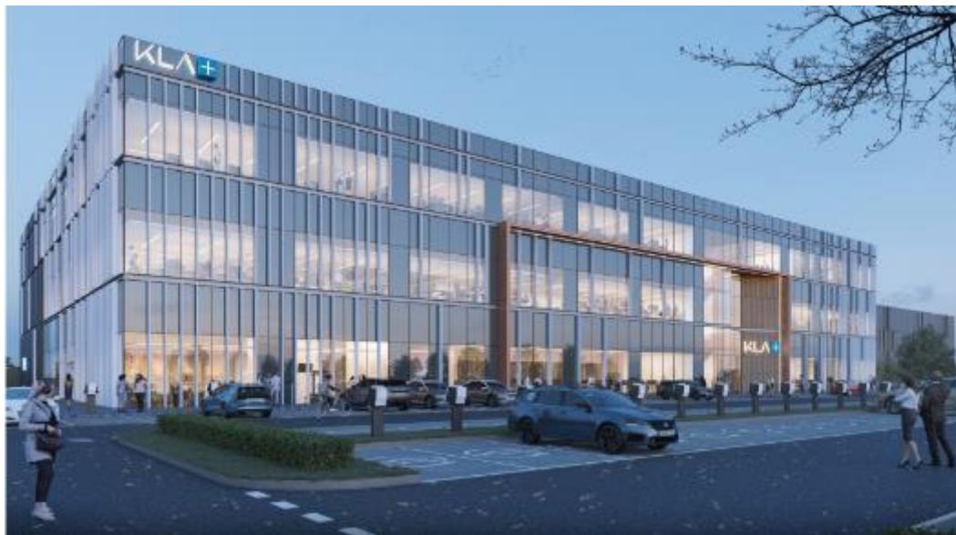
FIGURE 5: RESEARCH AND DEVELOPMENT FACILITY AT PLOT 1 AND 5, IMPERIAL WAY (EM1(i))
